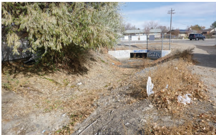
Figure 2- Former Utah Lake Distribution Canal channel looking northeast
