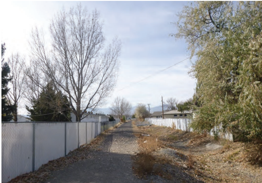
Figure 1- Former Utah Lake Distribution Canal channel looking southwest
